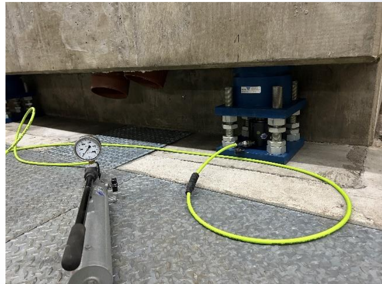
Installation of Spring Elements / Lifting of the Foundation
