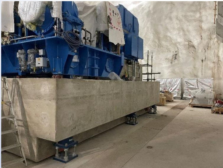
Installation of Spring Elements / Lifting of the Foundation
